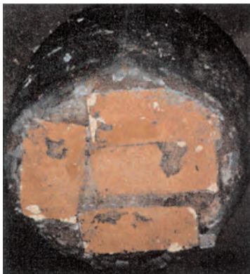
Example of brick being used instead of a stand.
