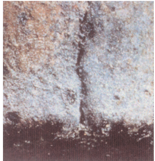
Bursting type crack from frozen heel of metal.
