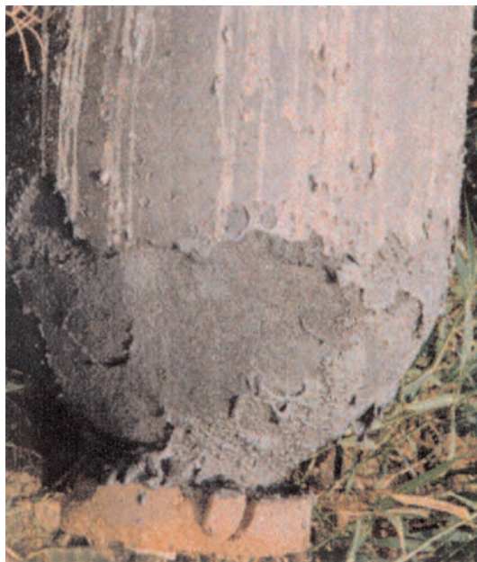
Severe crucible body deterioration caused by flame impingement as a result of a poor fitting stand.
