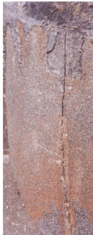
Top edge vertical cracking due to tight fitting grip-brick.
